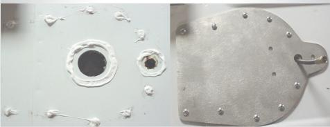
**5** Apply sealant to holes and attach base using the included hardware.
